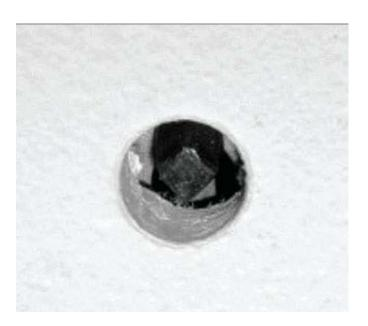
7. Drill a 1/2" diameter hole in the ceiling location that lines up with the centerline of the cable. (23/32" [18mm] from stud). Install ceiling drywall.
