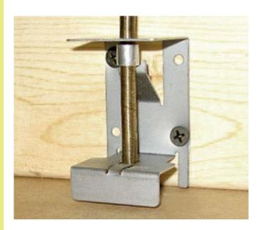
6. Attach the mounting bracket to the structural member so that the bottom of the bracket is flush with the underside of the ceiling.
