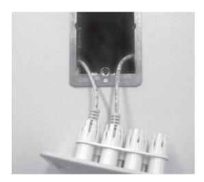
b. Route all connectors through the wall opening (paying attention to identify the connectors by location). Push connector into designated wall plate port until it snaps into place.
