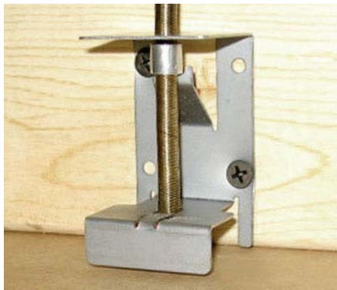
6. Attach the mounting bracket to the structural member so that the bottom of the bracket is flush with the underside of the ceiling.
