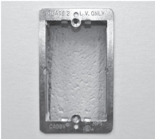
a. Use attached caddy instructions to prep the wall opening and install the mounting plate.
