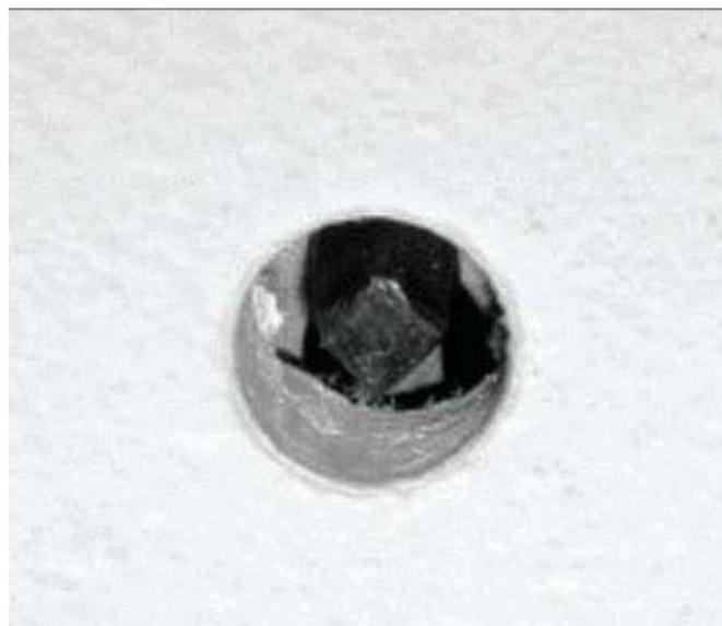
7. Drill a 1/2" diameter hole in the ceiling location that lines up with the centerline of the cable. (23/32" [18mm] from stud). Install ceiling drywall.
